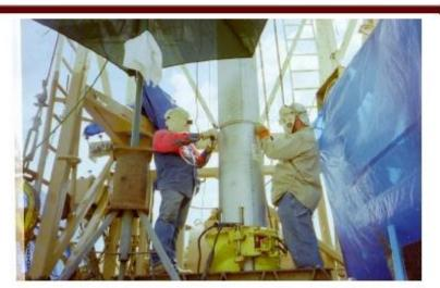
Welding and Fabrication of Duplex Stainless Steel
